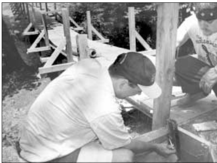
Patrick Moore, left, and Adam Lawson work to install an upright support for one of the new bridge rails. Both are from Allen Memorial UMC, Cleveland District. ☉
